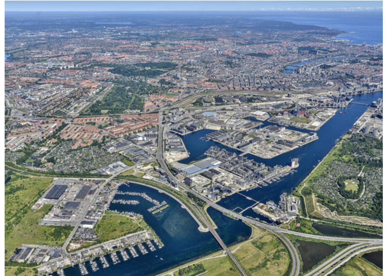
The new metro line to Sydhavn will consist of five new stations from Fisketorvet to Ny Ellebjerg.
