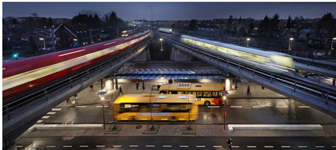
The Flintholm Station traffic hub is where buses, S-trains and metro trains intersect.
